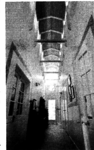
ABOVE AND BELOW: Clerestory roof is as dramatic inside as it is outside. Double glazing holds warmth in.
