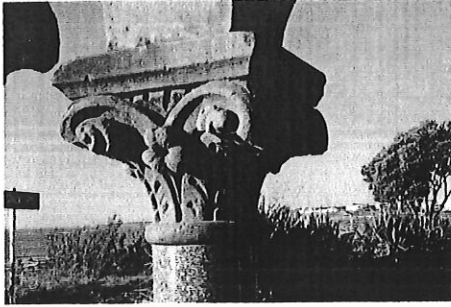
7 NE capitals showing alveolisation cracking and volute damage
