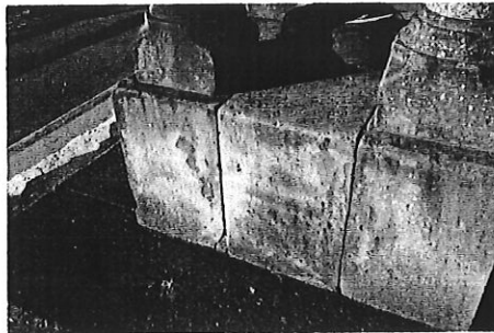
9 West showing plastic repair, pitting and skin damage to base
