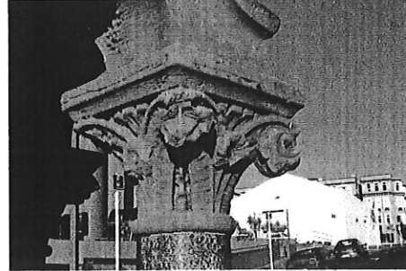
2 SW capitals showing volute damage and alveolisation
