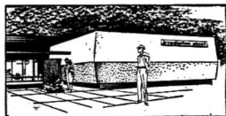
This concrete building, with walls up to 5 ft. 6 in. thick, will contain the energy source, Cobalt 60, in Tasman Vaccine's Gamma Sterilisation Plant.
