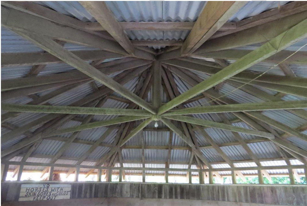
The exposed internal roof structure
