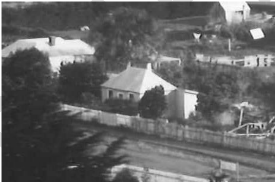
Detail from undated, circa early-mid 1890s image showing rear-hipped gable removed, and present lean-to in its place. Puke Ariki, A.3.297
