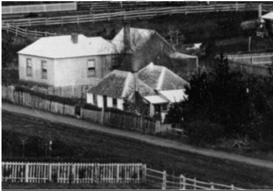
Detail from photograph of New Plymouth taken between late-1880 and late-1883, showing cottage before removal of rear hipped-gable section. Alexander Turnbull Library, Fred B. Butler Collection, PAColl-4127-01
