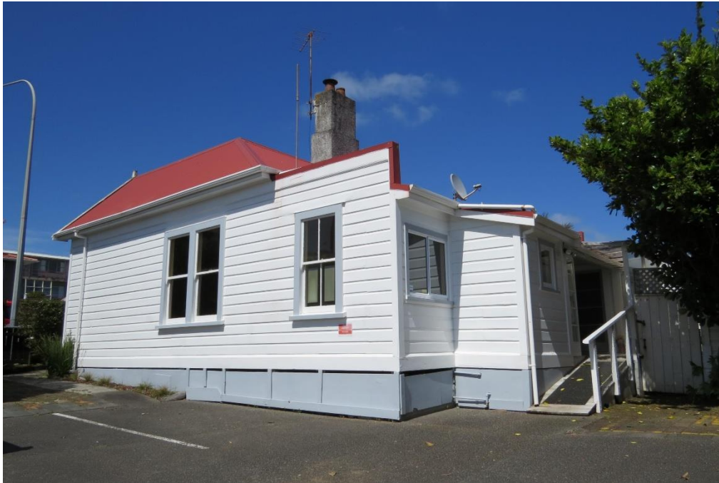
View of north-eastern elevation showing lean-to parapet wall
