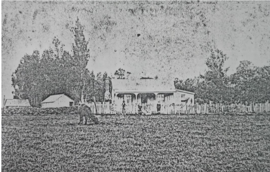
Circa 1885 view of Soffe House before gable addition, from Fraser, D. P. (1989). Waitara . D. P. Fraser, Waitara, source of original photograph unknown.
