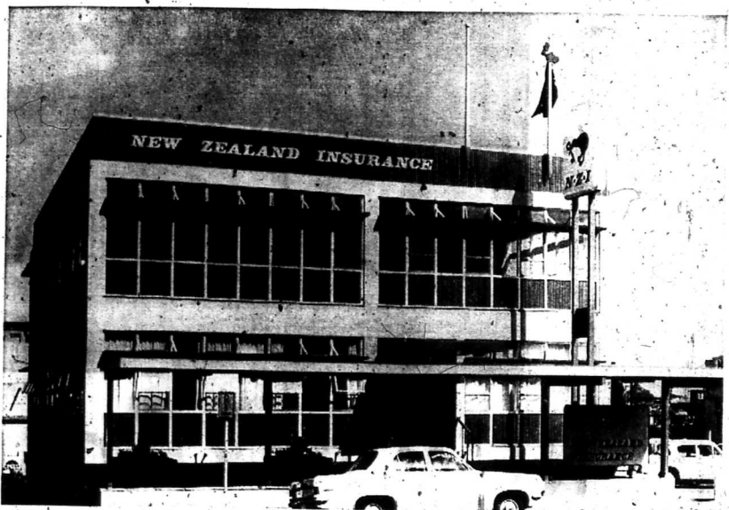
THE NEW ZEALAND INSURANCE CO.'s new $100,000 New Plymouth branch office building which is to be officially opened tomorrow by the company's chairman of directors, Mr. A. G. Wilson (Auckland). The main entrance is in Currie St. opposite the Chief Post Office.
