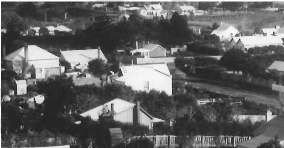
Detail from circa early-mid 1890s (pre-1895) view of New Plymouth from Fort Niger showing rear and SE elevation of 94 Lemon Street; 92 and 96 Lemon Street are yet to be constructed. Puke Ariki, A.3.297.
