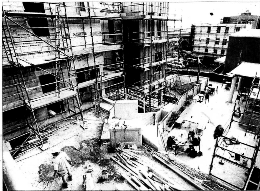
Coffee courtyard: The King and Queen Hotel Suites entrance is designed to allow foot traffic to flow into the Ozone Coffee Roasters courtyard pictured.
