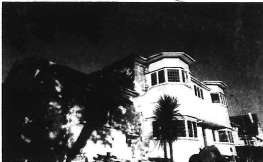
WORK IN PROGRESS: The hotel in Brougham St, New Plymouth.
