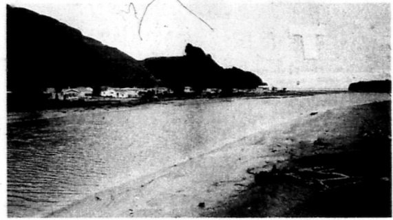
ABOVE: The baches at Tongaporutu, which must be gone by 2005.
