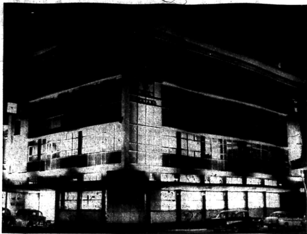
SPOTLIGHTING is used effectively at night to bring out the architectural features of the handsome new Bank of New Zealand premises in Devon and Brougham Streets, New Plymouth. The lighted interior indicates the banking chamber on ground floor and mezzanine floor, above, in which there are offices for the bank manager, security department and staff rooms. The top storeys are to be leased to tenants as offices.
