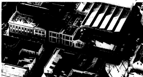
An aerial view of the Taranaki Newspapers Ltd complex on the corner of Currie Street and Powderham Street, New Plymouth before the old Herald site was demolished.
