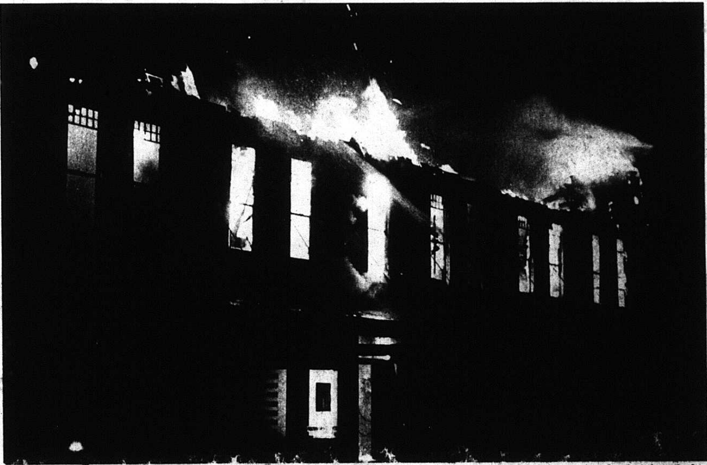
At the height of the fire in an old wooden block on Egmont St, New Plymouth, firemen had to battle to stop flames spreading to adjoining buildings.
