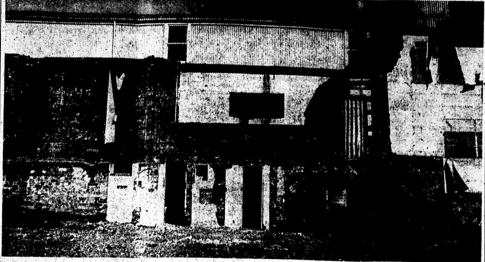
THE REMAINS of the old Imperial Hotel as they were when the demolition contractor left the site today. The two open doorways provided access from Devon St to lavatories.
