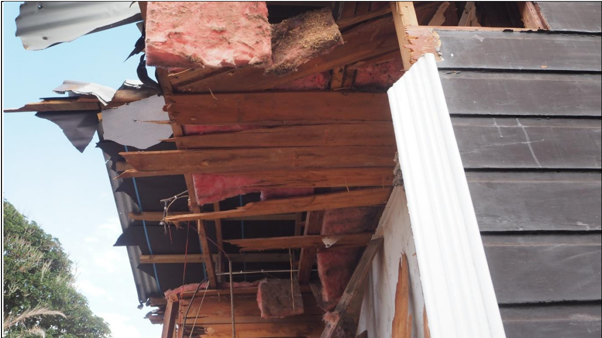
Figure 24: Undressed ceiling boards noted during demolition. Image: Ivan Bruce, 2017.
