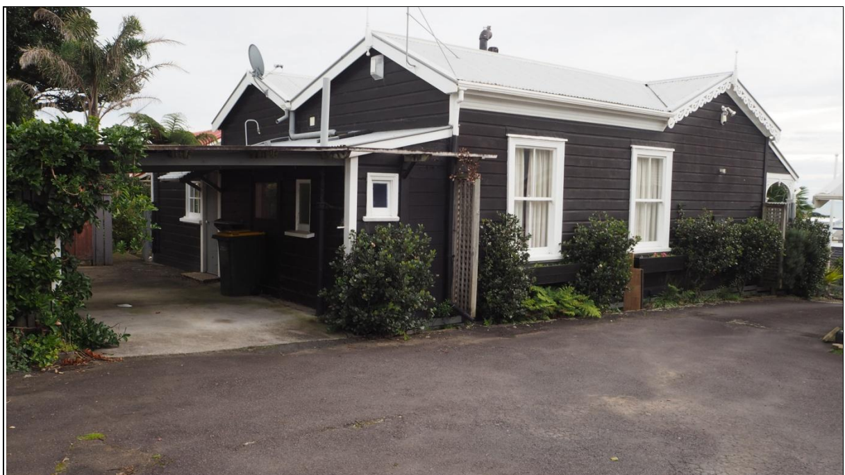
Figure 8: Photograph of the eastern elevation. The four-pane sash windows, decorative barge boards and rusticated weatherboard cladding are all original. Image: Ivan Bruce, 2017.
