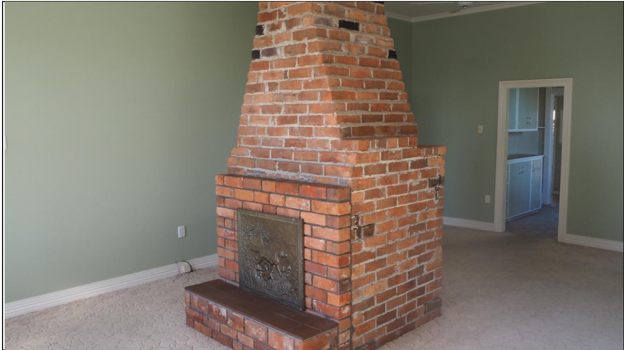
Figure 34: The double fire place. A dividing wall between what was most likely the dining room and the kitchen room had ben removed sometime prior to 1986 renovation Image: Ivan Bruce, 2017.
