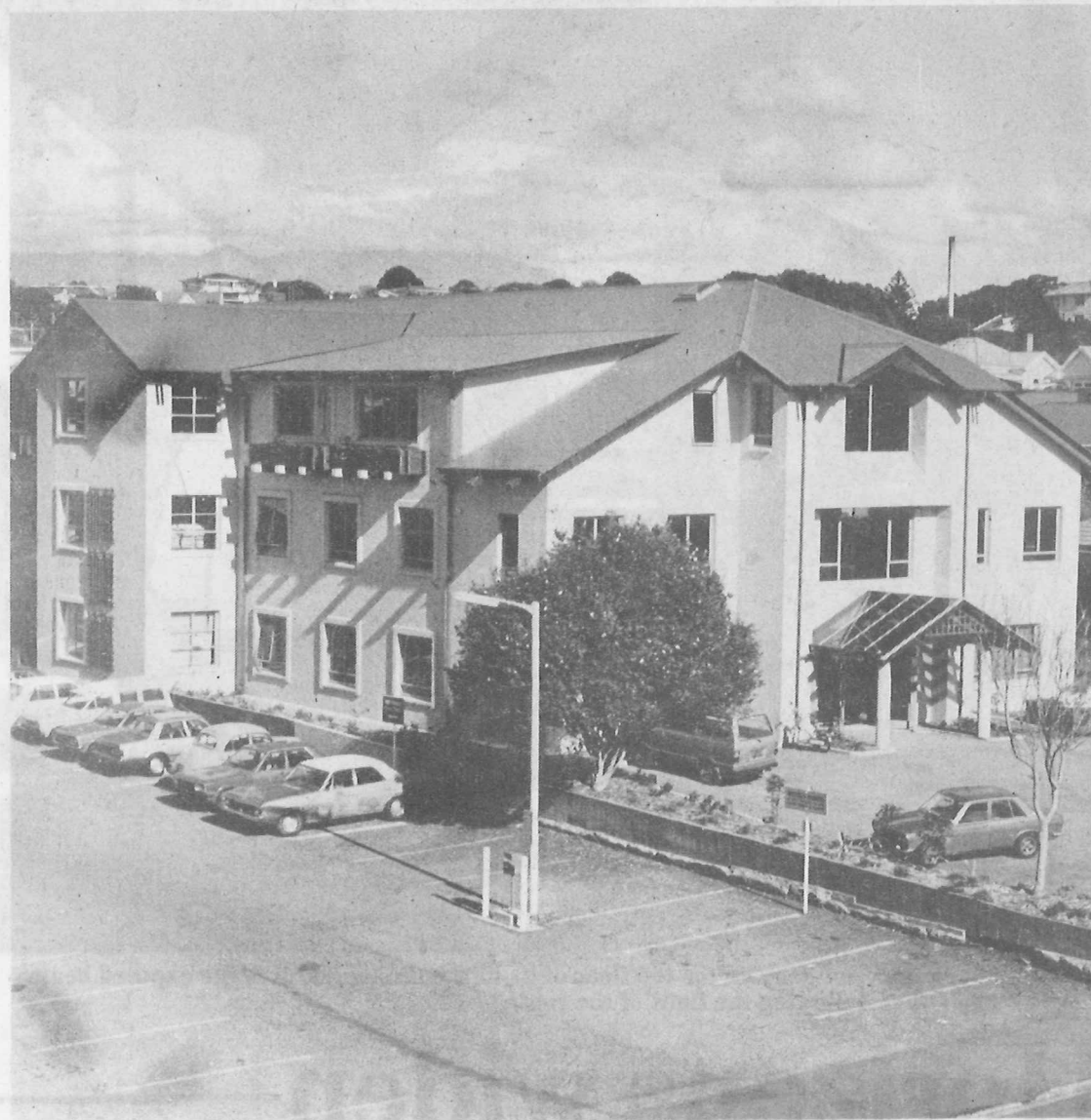
The unusual lines of Arthur Young House provide a bridging effect visually between the more residential designs of the buildings on one side and the conventional aspect of other New Plymouth commercial buildings on the other side and across Powderham St. The three floors of the city's newest building accommodate the New Plymouth office of Arthur Young and Company on the top floor and part of the second floor, optometrist J. S. McKinnon on the remainder of the second floor and Shell BP and Todd Oil Services on the ground floor.
