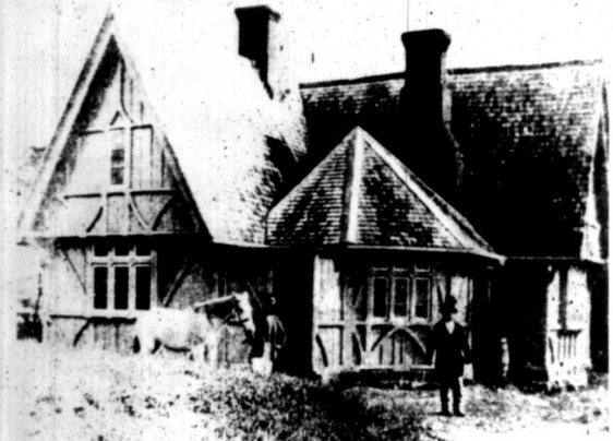
The Gables, when built...
