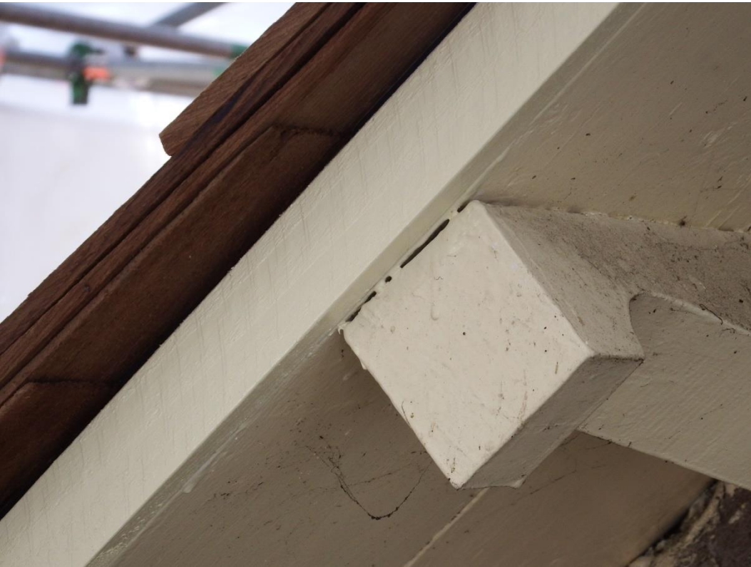
Timber edge conceals plywood
