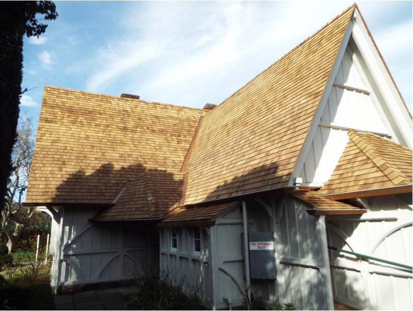
Completed Works August 2017
