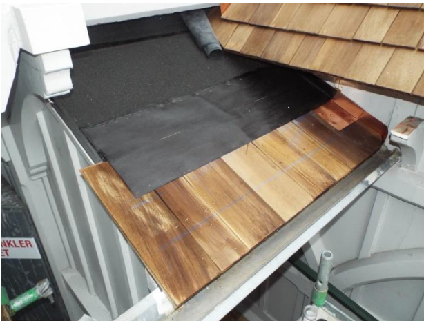
Building paper between each layer of shingles
