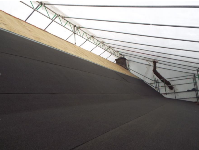
Peel & stick over plywood
