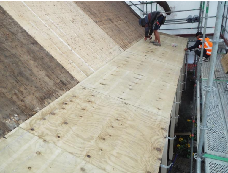
Plywood overlaid on sarking
