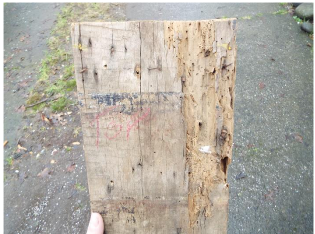
Removed timber sarking
