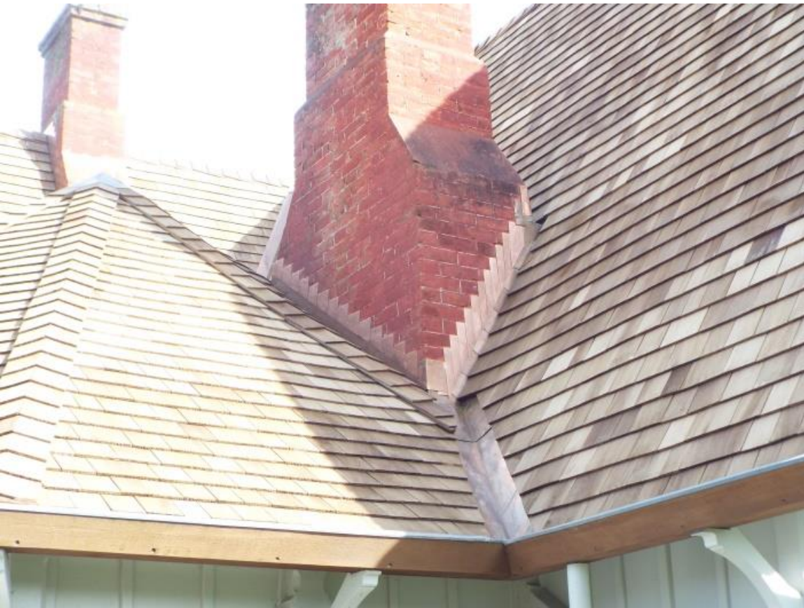
Completed step flashing and copper valley
