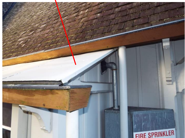
Metal roofing on particle board substrate replaced with shingles on plywood
