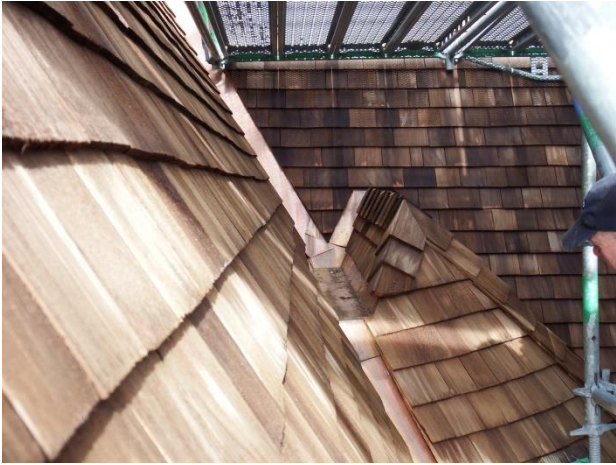
Intricate copper valley behind conical roof
