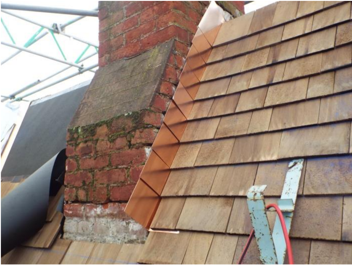
Chimney step flashings
