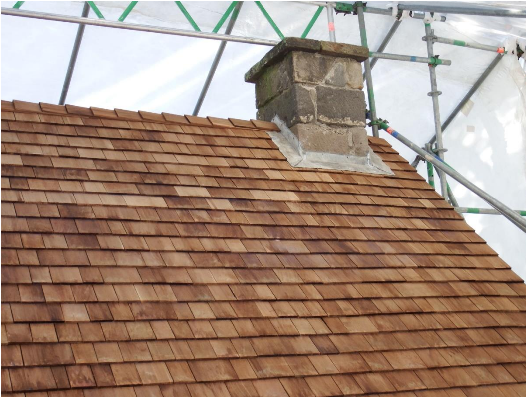
Existing lead flashing retained
