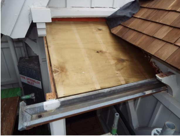
Plywood laid for peel & stick membrane to be applied
