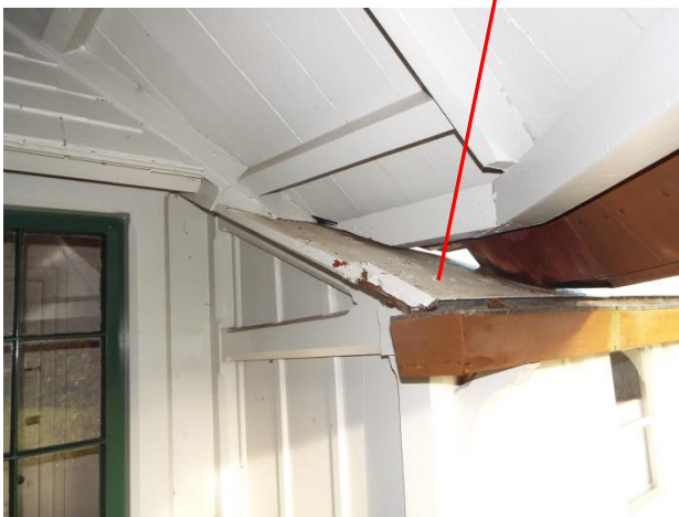
Metal roofing on particle board substrate replaced with shingles on plywood
