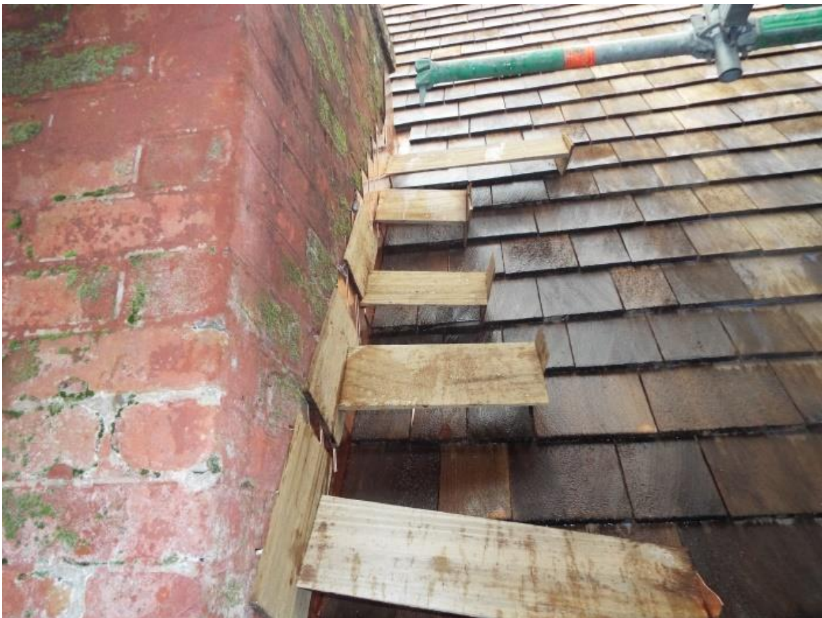
Chimney step flashings
