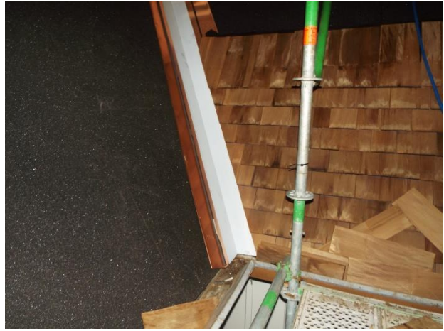
Copper valley flashing
