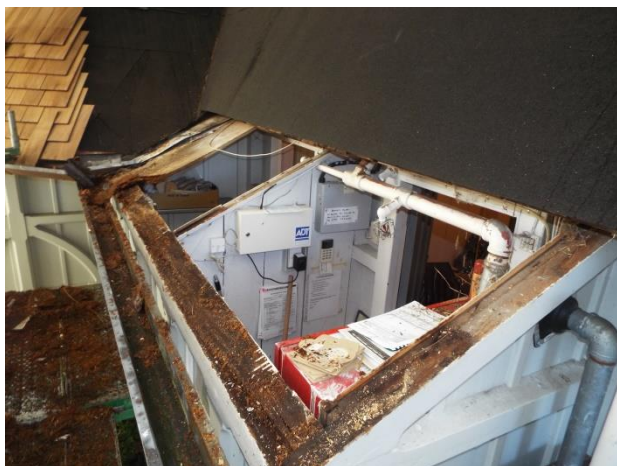
Rotted particle board substrate removed.
