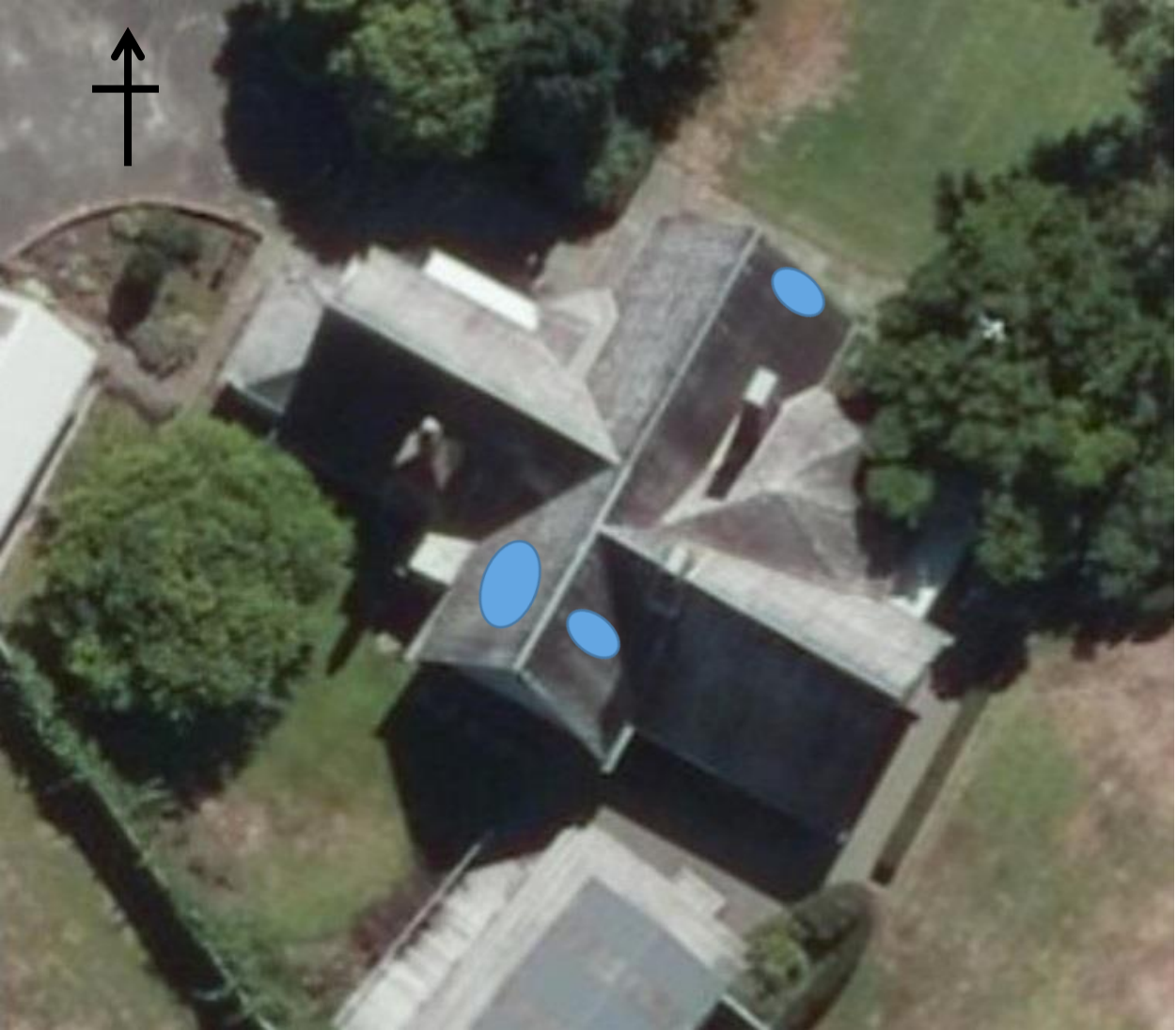
Ariel view showing areas of ceiling sarking replacement
