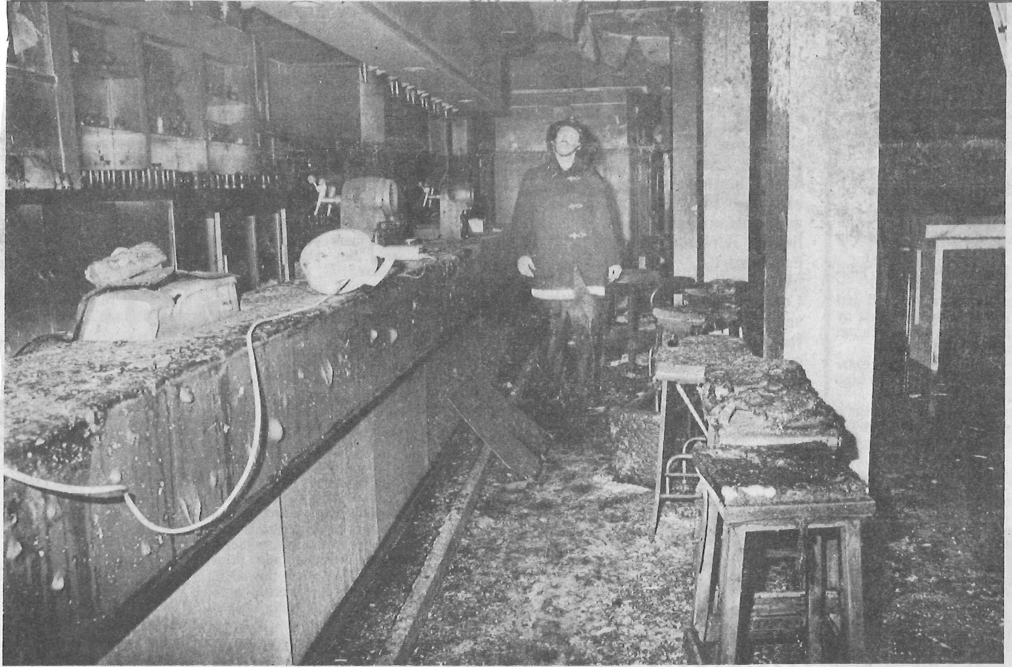
New Plymouth Fireman Chris Haunton surveys the burnt-out shell that was the Royal Hotel public bar.
