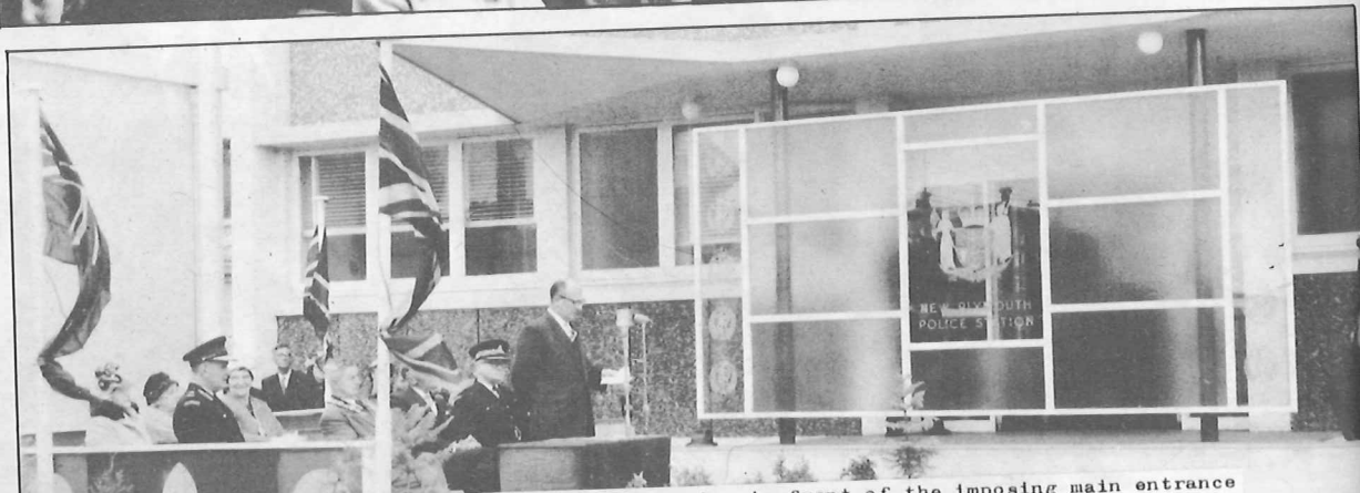
Mr Eyre making his official address on the dais, in front of the imposing main entrance
