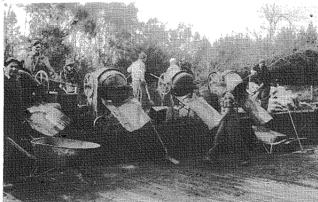
Concreting floor of the pool.
