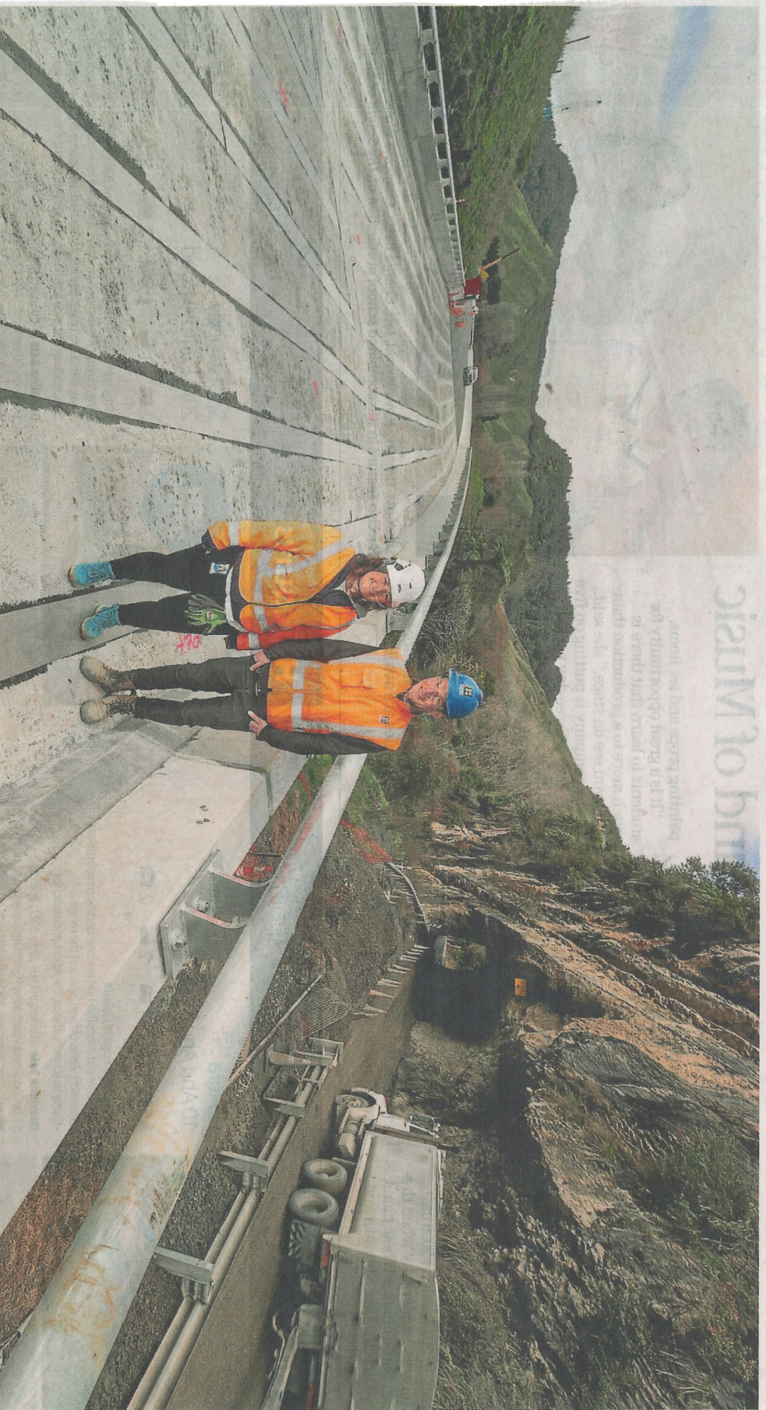
Waka Kotahi NZTA regional infrastructure delivery manager Jo Wilton and Fulton Hogan project manager Blair Jacobs on the new bypass bridge beside the old tunnel access. SIMON O'CONNOR/STUFF
