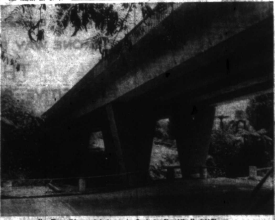
New Plymouth's new viaduct, spanning Carrington St and the Hikutakaho Stream.
