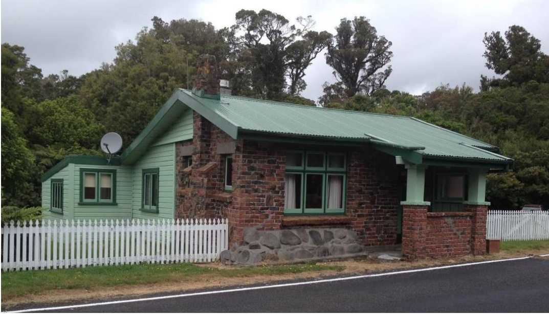
Figure 10: View of northern and western elevations showing kitchen at far left (in former laundry), Elizabeth Pishief, 31 January 2015 (cropped image)
