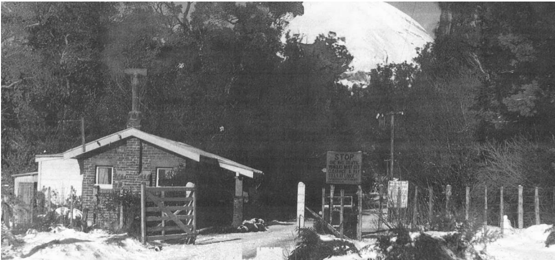
Figure 7: Rahiri Lodge circa 1930. Note the lean-to at the rear (likely the bathroom), which is in the position of the concrete slab in the floor today. There is also a structure just discernible behind the ‘Stop’ sign which may be a telephone box. 113 Image provided by Dave Rogers, Department of Conservation Ngāmotu Area Office, reproduced in Pishief, 2015, 9.
