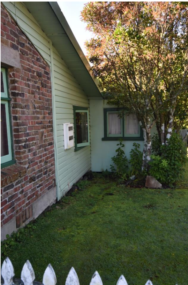
Figure 13: Looking east along southern elevation showing original 1929 'clinker brick lodge', 1937 weatherboard addition and third bedroom in asbestos board addition from circa 1946-1948
