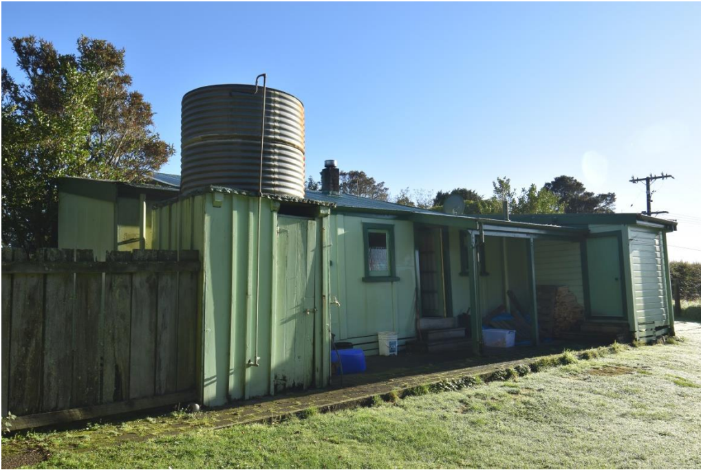
Figure 12: Rear (eastern) elevation of Rahiri Lodge showing tank with pump/storage shed, back door, verandah and storage shed door at far right
