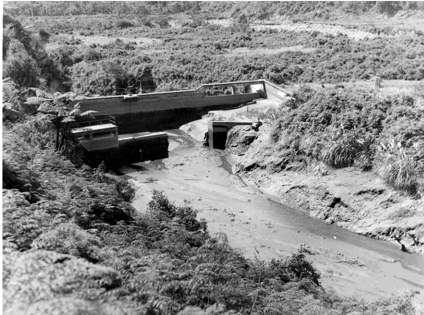
1914 (closest) and 1917-18 Dams on the Māngamāhoe Stream during a draining of the lake about 1950. Waiwhakaiho River is in the distance.
