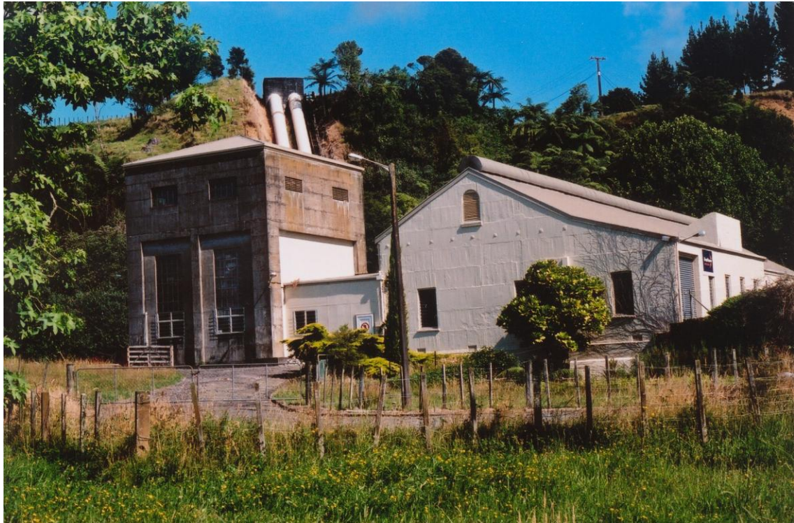
Mangorei Power Station - 2007
