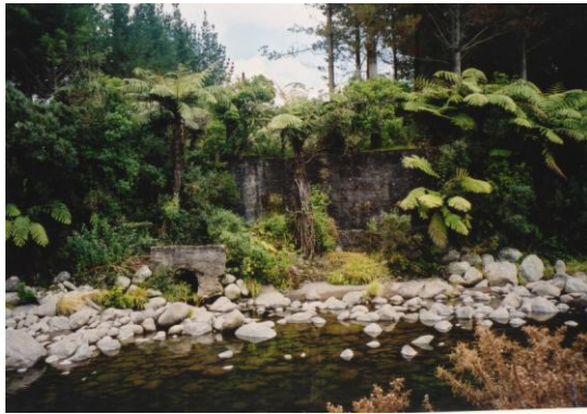
1906 Intake, Waiwhakaiho River – 2002
