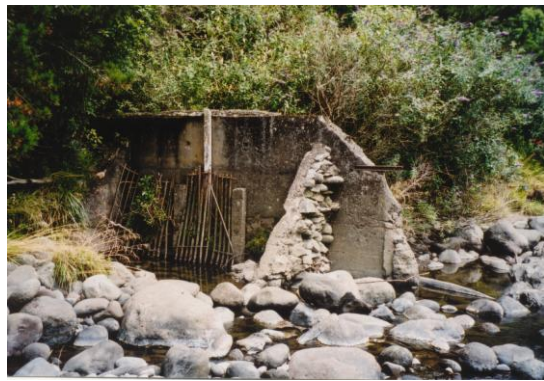
1914 Intake, Waiwhakaiho River - 2002
