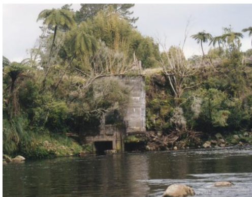
1923-24 Surgetank and outflow - 2002
