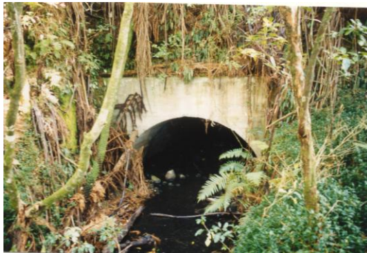
1914 Race-tunnel to dam
