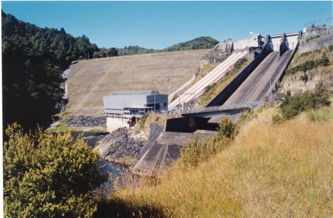
Pātea Dam, Penstocks and Generating Station
