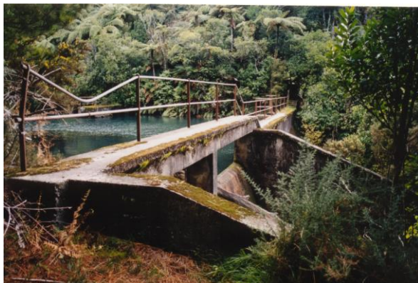
1917-18 Low Head Dam, Māngamāhoe Stream - 2002
