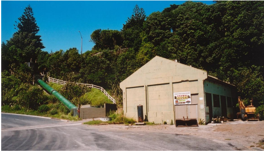
Opunake Power Station - 2007
