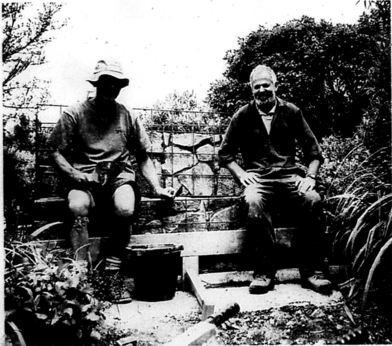
BE SEATED: Hawera alpine enthusiasts Dave McNair (left) and Kevin Dwyer take a spell during the construction of the new Sir Edmund Hillary seat above Dawson Falls. Photo: SUPPLIED
