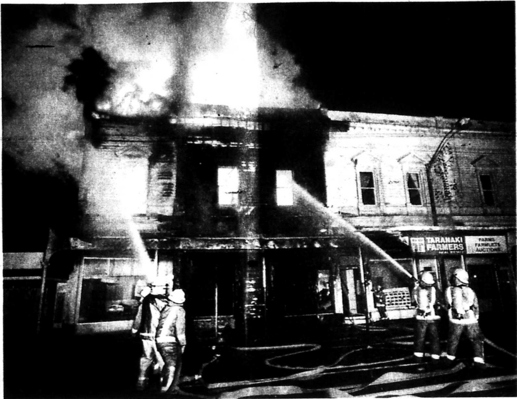
BLAZING AWAY: Firefighters battle the blaze in one of Inglewood's most historic landmarks in the town's main street early yesterday morning. The fire was contained in the western half of the wooden building. Photos: ADRIAN MALLOCH
